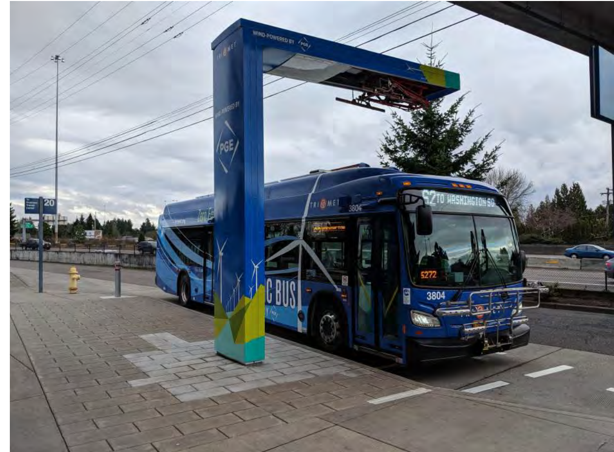
TRIMET SUNSET TRANSIT CENTER - BEB FAST CHARGER
