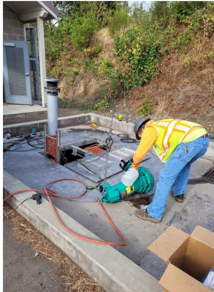
Maintenance on S Ivy Pump Station
